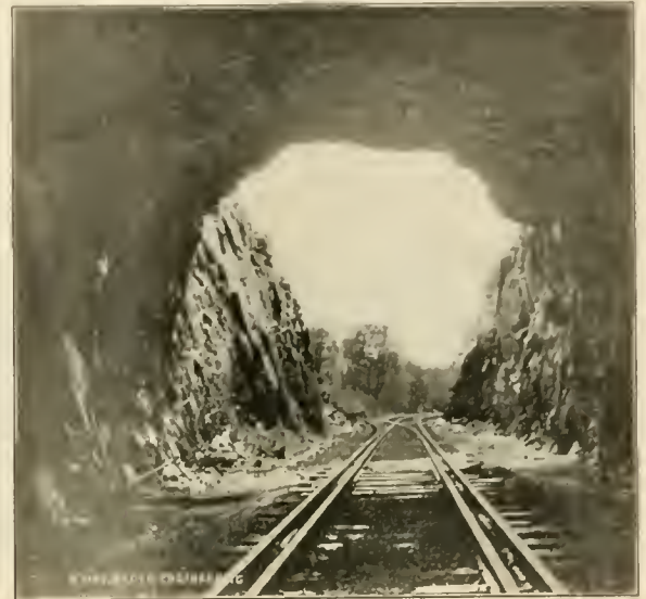
VIEW FROM INTERIOR OF OXFORD TUNNEL ON THE LACKAWANNA, SHOWING GAUNTLETED TRACKS.
